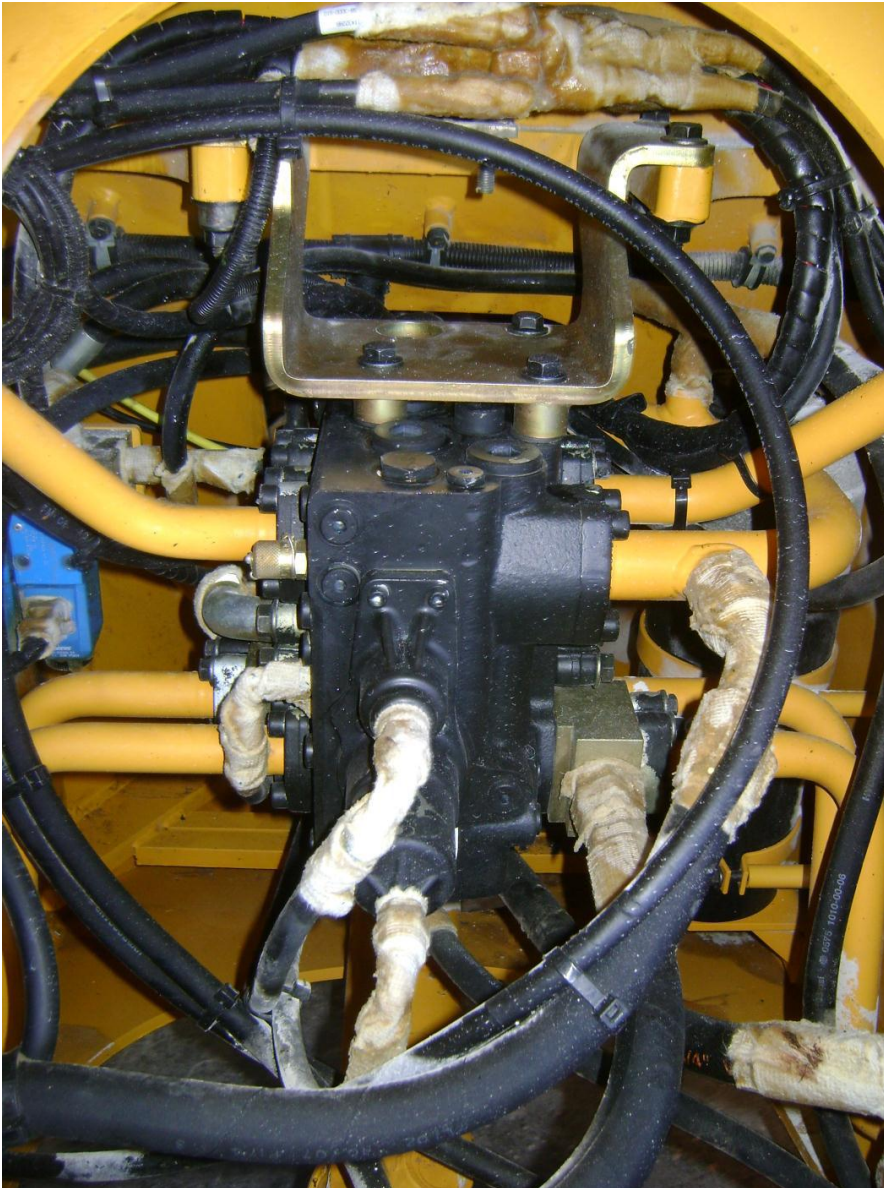
Figure 8: Loader washed hot water ready for treatment
